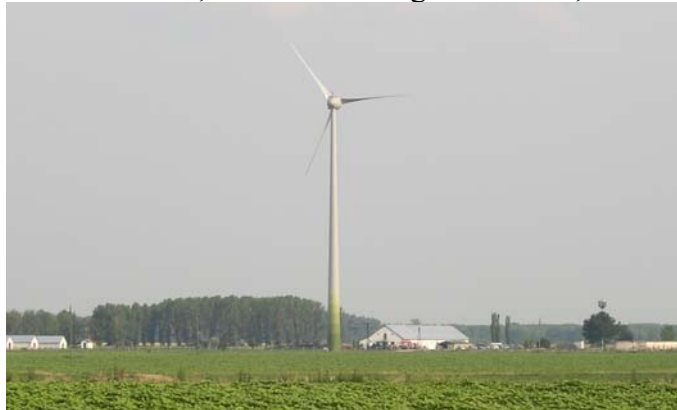
Fig. 3.1 Wind generator at village Erk (Enercon E-48, 800 kW, 76 m) (source: author's shot)
