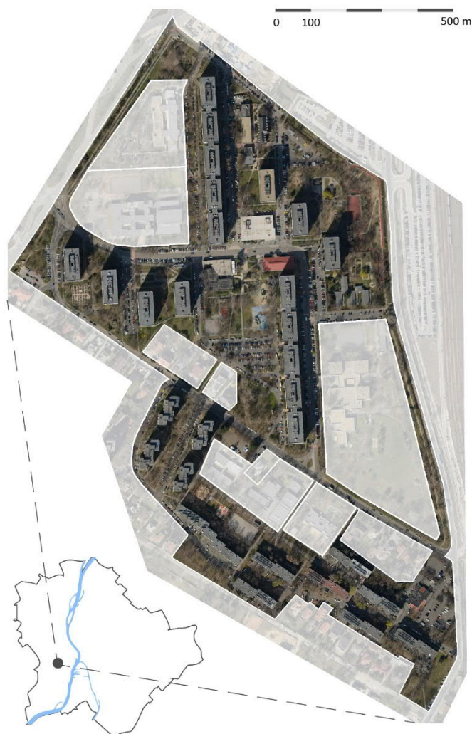
FIGURE 33: LOCATION AND SATELLITE PICTURE OF THE ÓRMEZŐ HOUSING ESTATE
