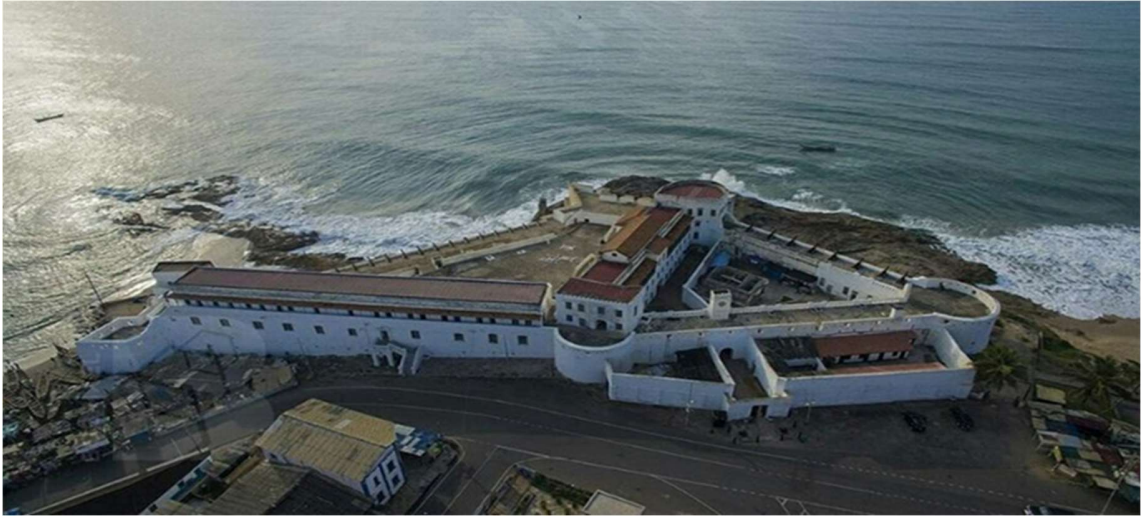
Figure 7: Aerial view of Cape Coast Castle on the Atlantic Coast Source: GMMB, CAPE COAST, GHANA (2018).
